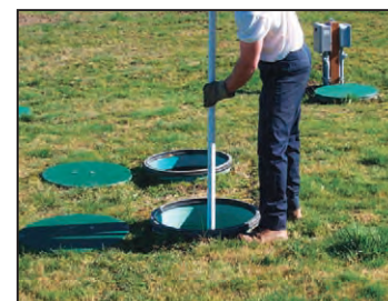
Septic tank inspection in progress
