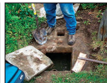
Septic tank baffle screen inspection in progress
